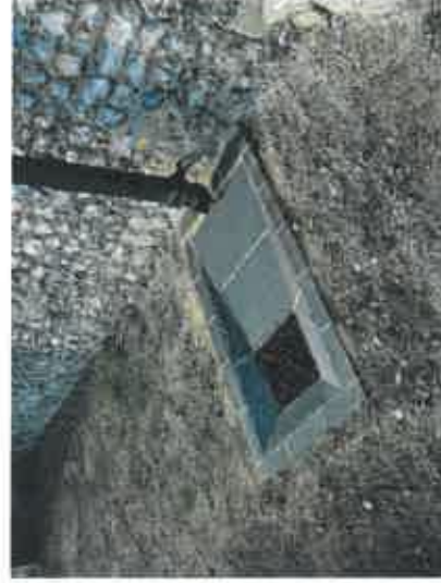
Hepworth 225mm x 400mm outlet with medium duty grating: Code RGP6 + Silt bucket IBP3. Remove fixing screws on grating. These gullies are available with a back inlet if the layout drawings and Works Schedule shows this to be required.
