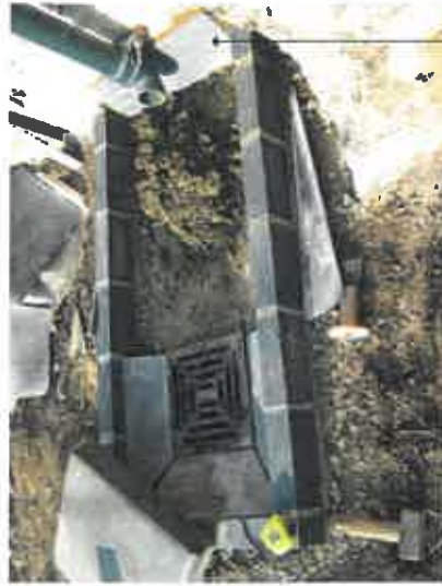
Slate up stand against wall to be one piece of slate.
